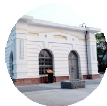
Water Metering Room
